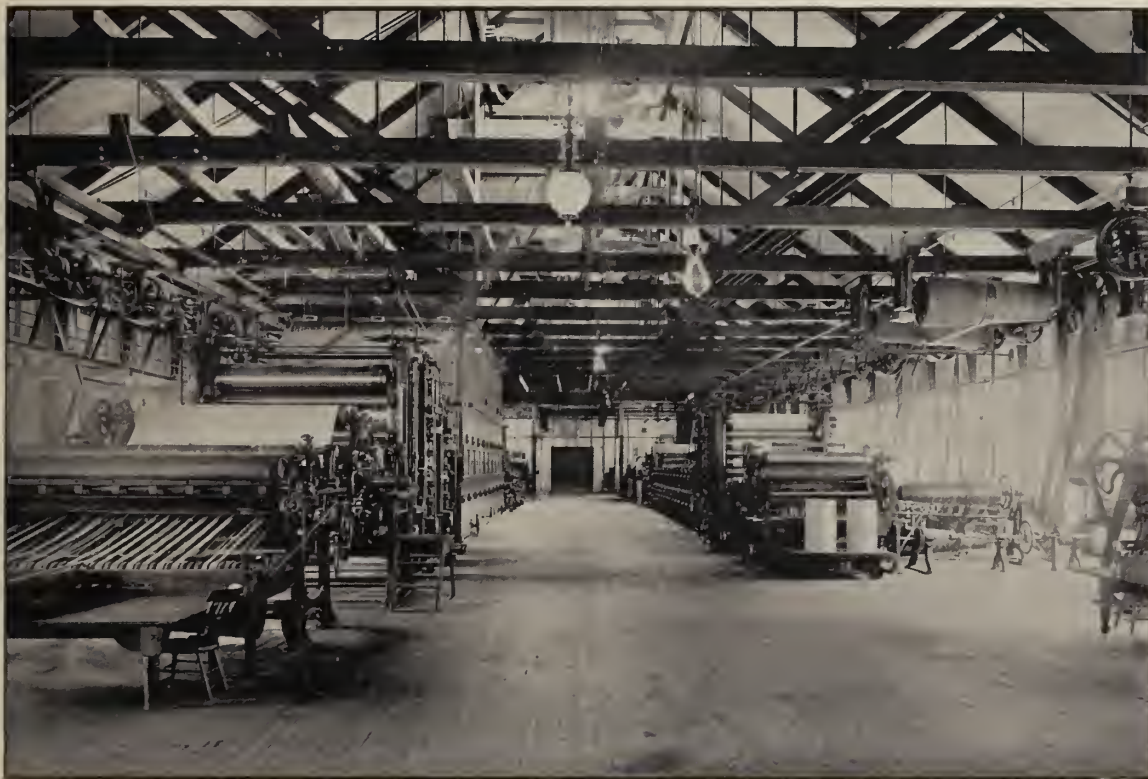
PAPER MACHINE ROOM OF THE HOLLINGSWORTH & WHITNEY CO.
